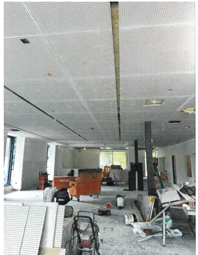
Progress photo level 1 children's wing
