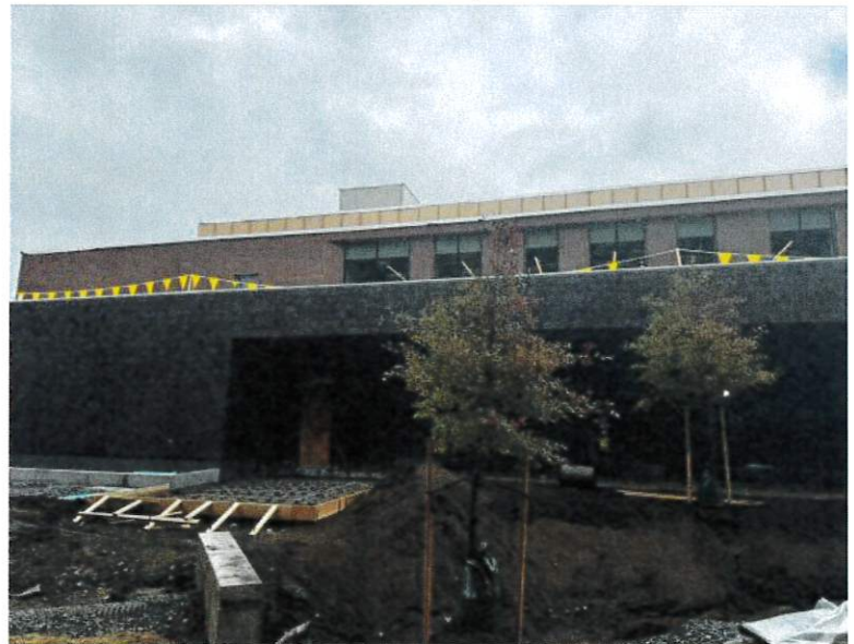
Progress photo south elevation siding
