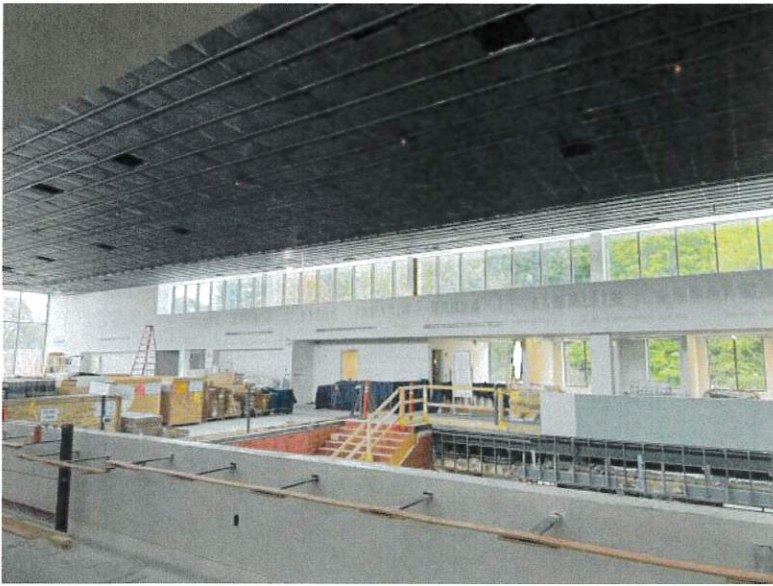
Progress photo level 2
