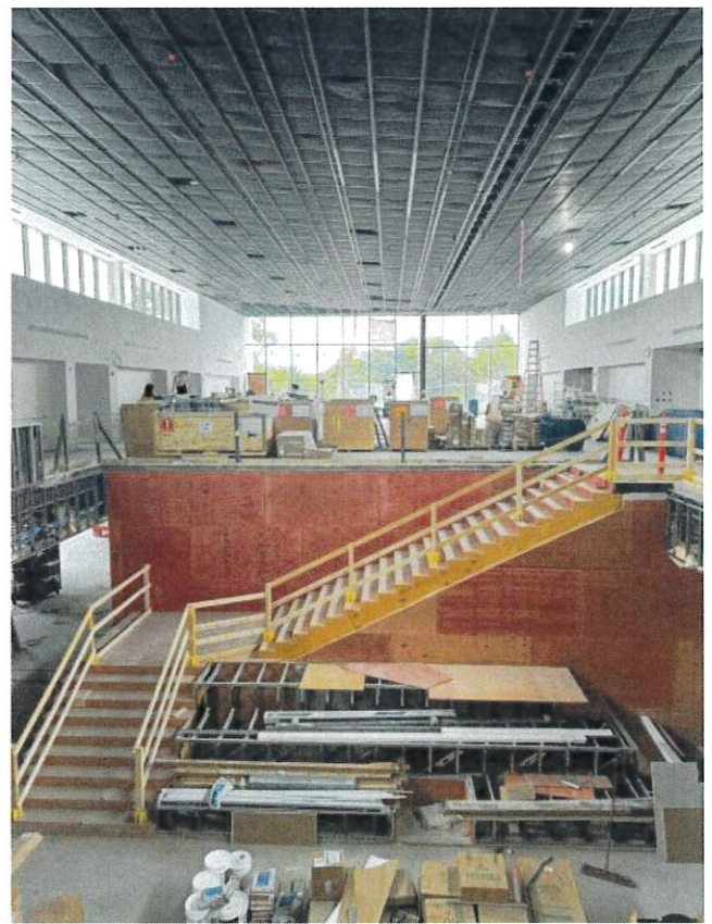
Progress photo grand staircase
