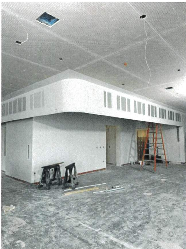
Progress photo level 1 children's wing
