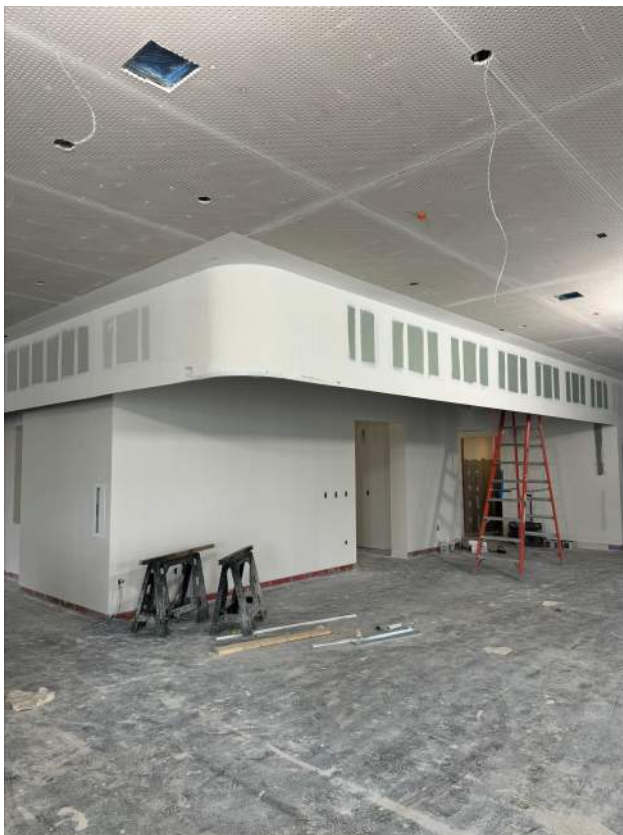
Progress photo level 1 children's wing
