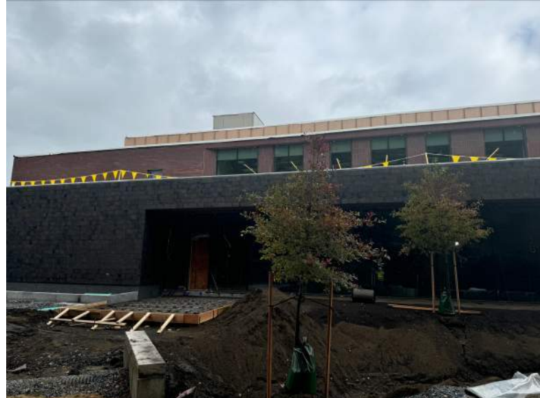
Progress photo south elevation siding
