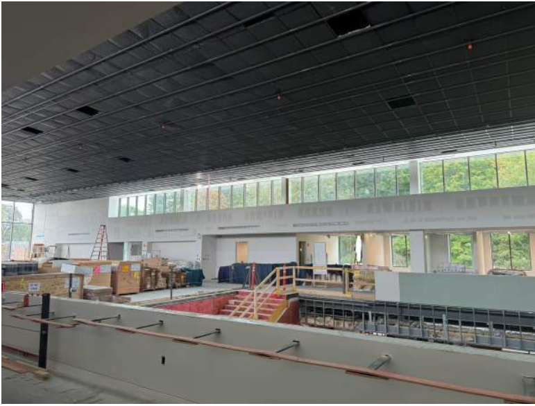
Progress photo level 2
