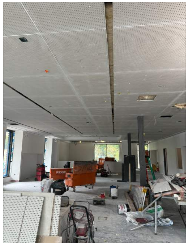
Progress photo level 1 children's wing
