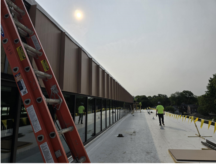
Installing imitation wood panels.
