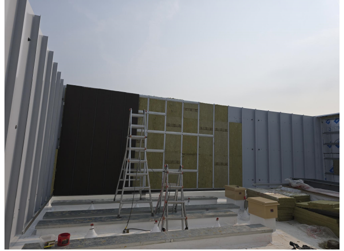
Installing metal panes at mechanical well.
