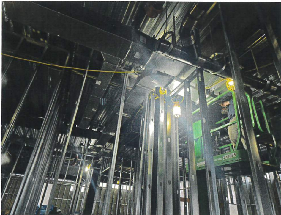
Hanging ductwork 1st level
