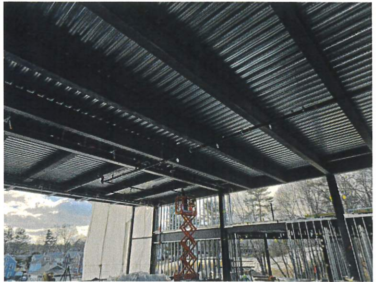
Installing fire protection piping
