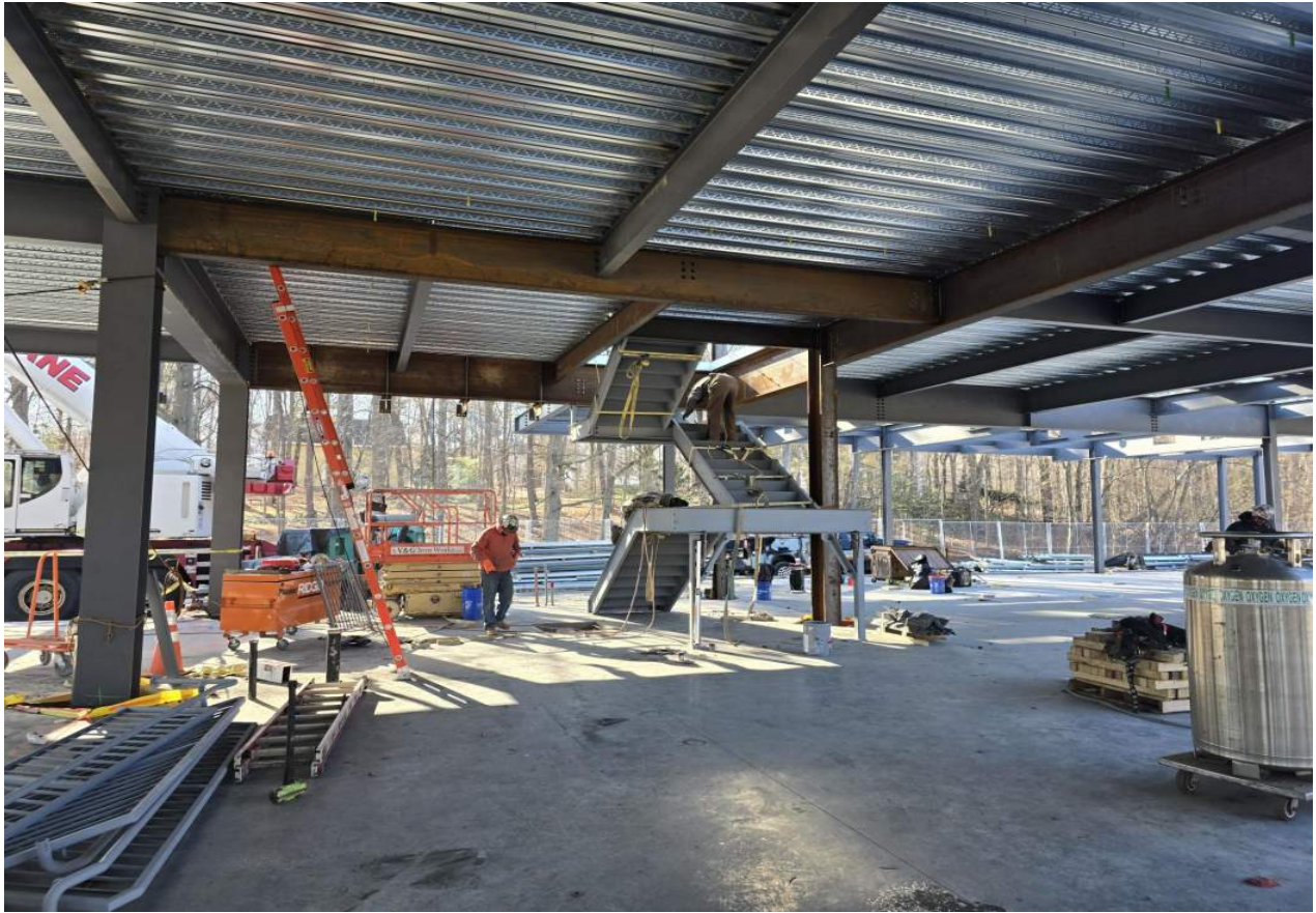
Staircase installation
