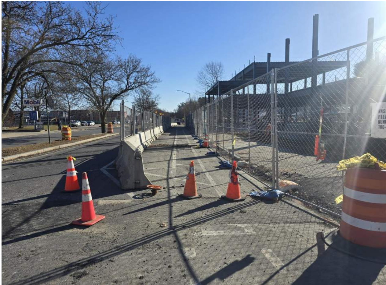
Temporary Sidewalk & Fencing
