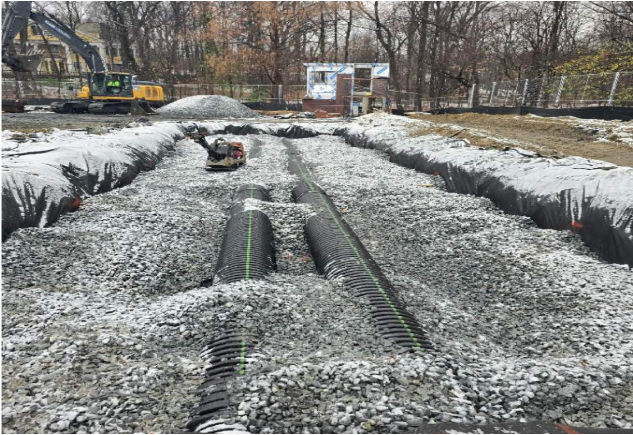
Drainage infiltration system install
