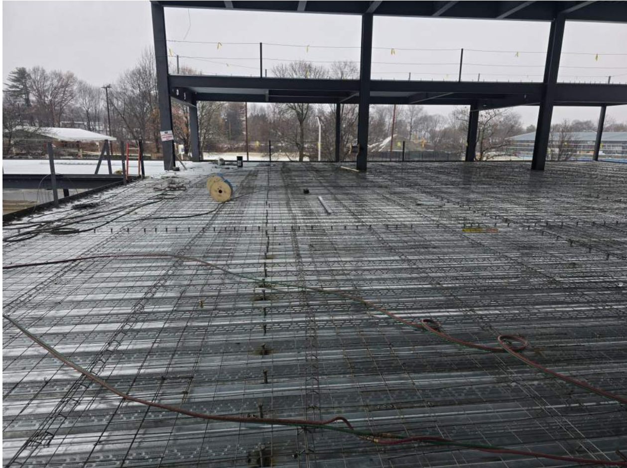
2nd level decking and WWF install
