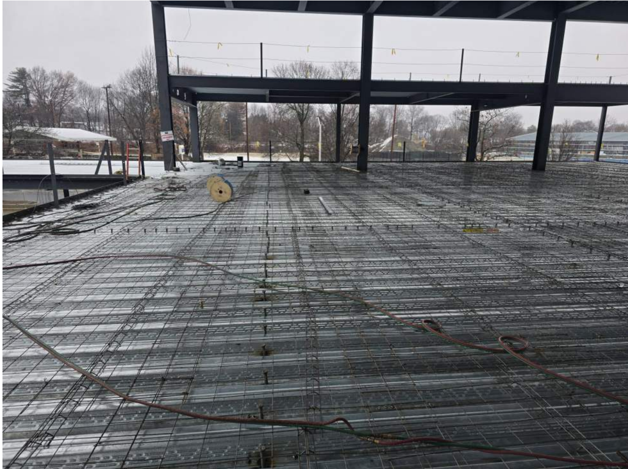
2nd level decking and WWF install
