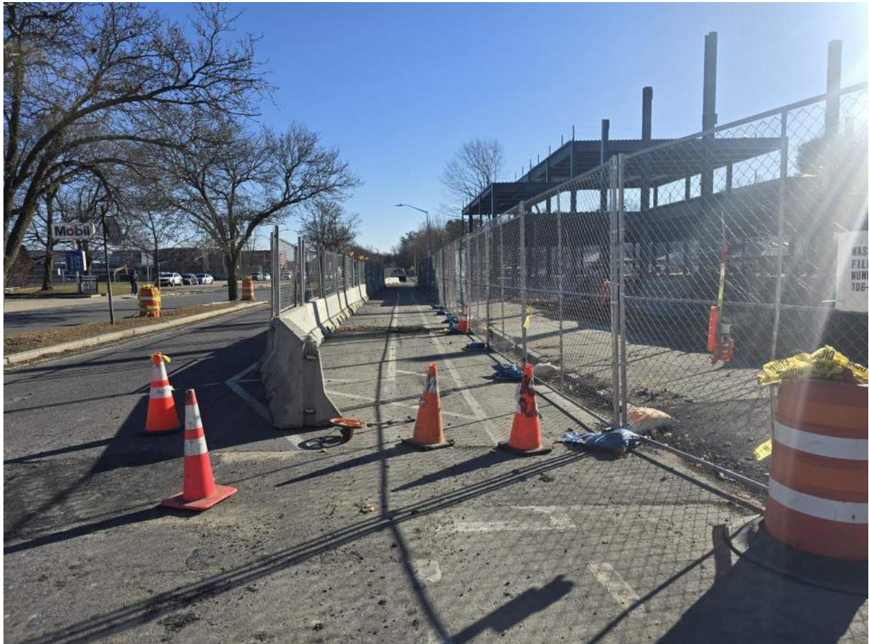
Temporary Sidewalk & Fencing
