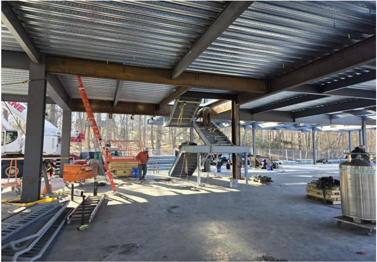
Staircase installation
