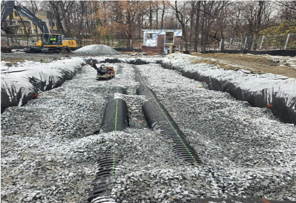
Drainage infiltration system install
