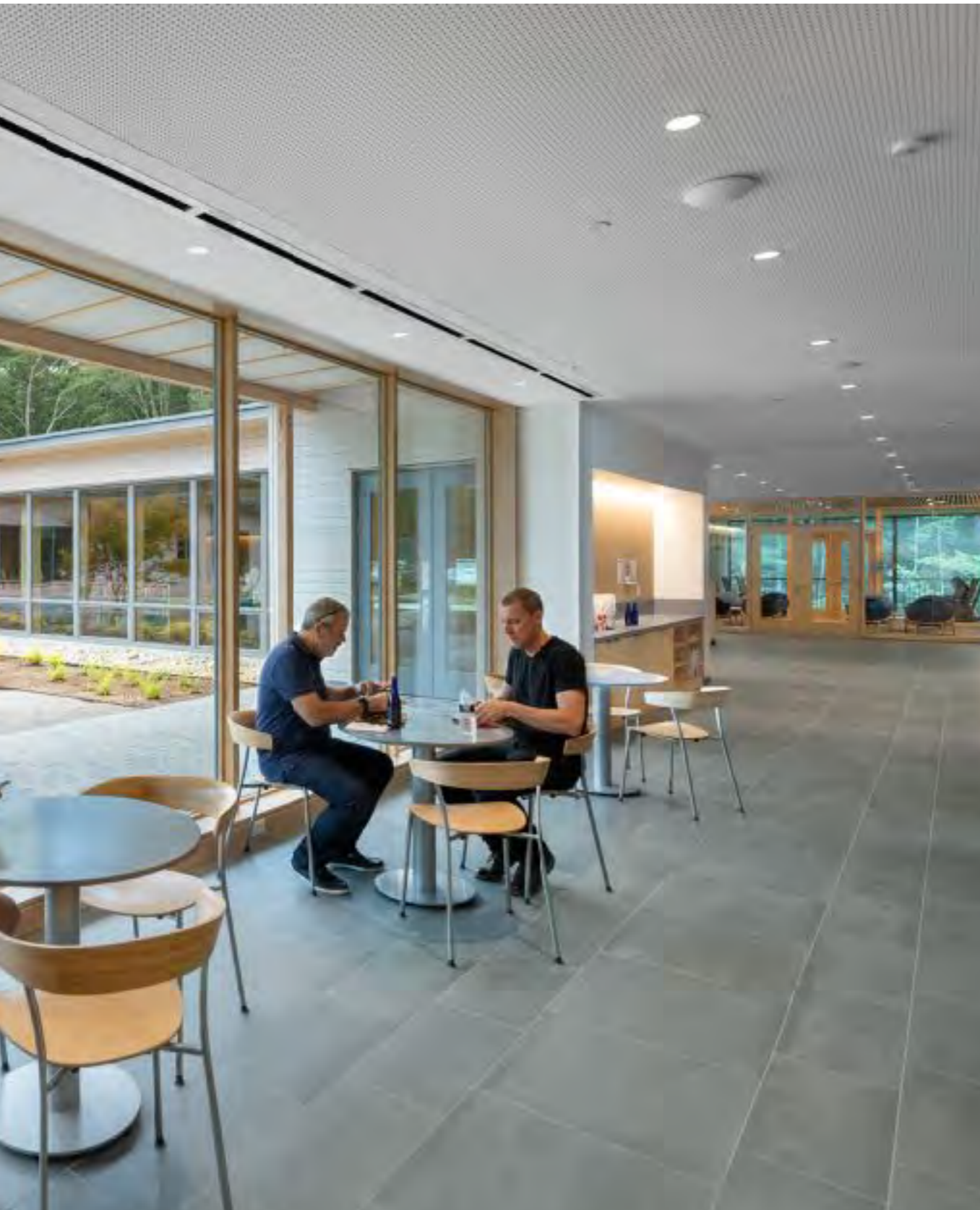
Perforated GWB Ceiling
