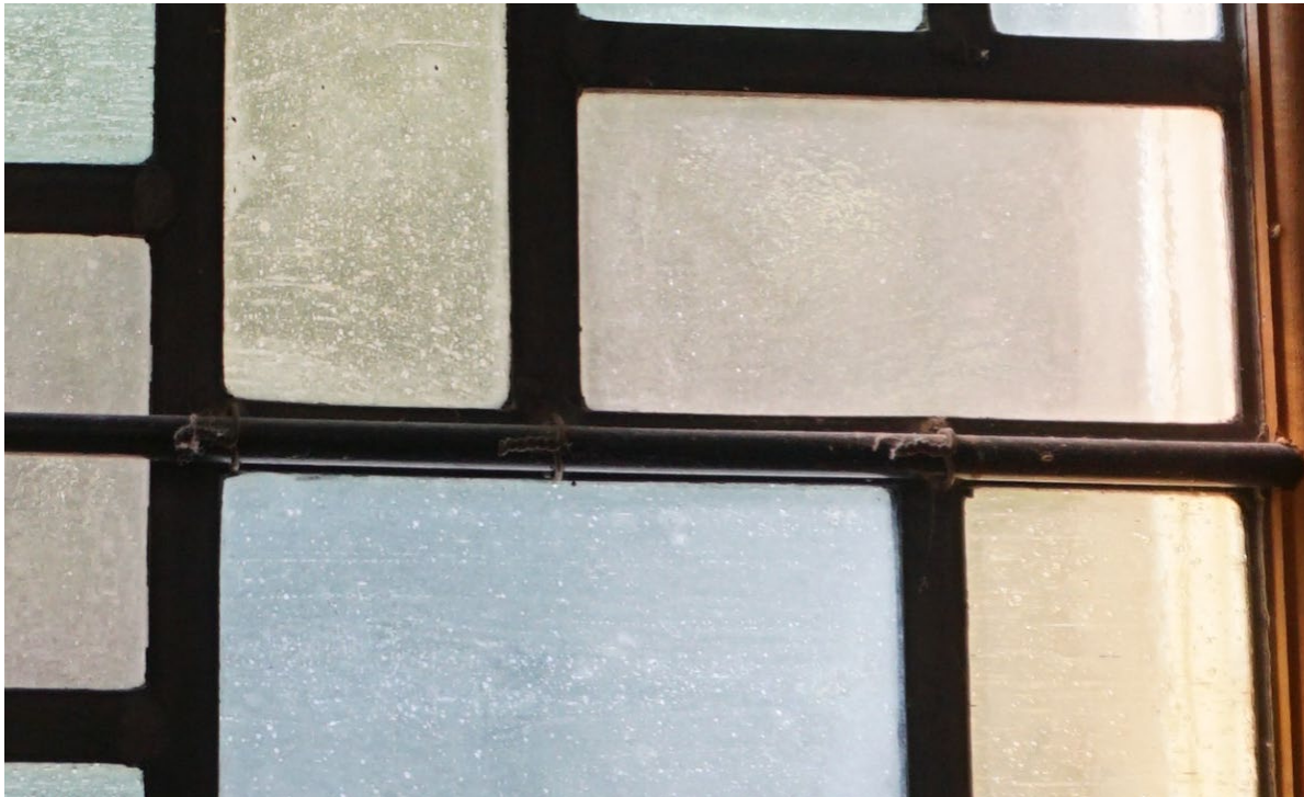
Figure 1. Wire ties connecting stained glass window to saddle bar. This is needed for stabilization, because the lead between each glass pane is very soft.
