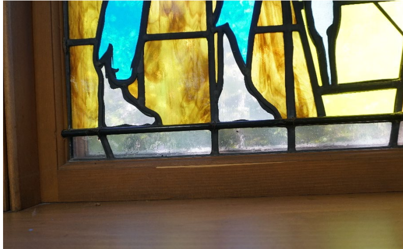
Figure 2. Crack in Tom Sawyer window sash.
