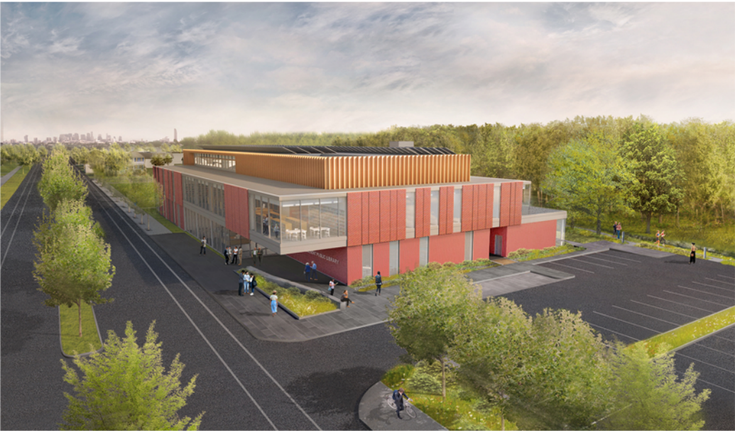
EX Aerial Northwest (REV 2022).jpg
