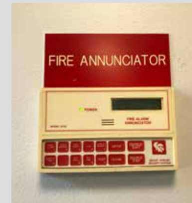
FIRE ALARM SYSTEM IS UNRELIABLE AND NEEDS TO BE FULLY REPLACED (WHICH IN TURN REQUIRES A NEW ELECTRICAL SYSTEM)
