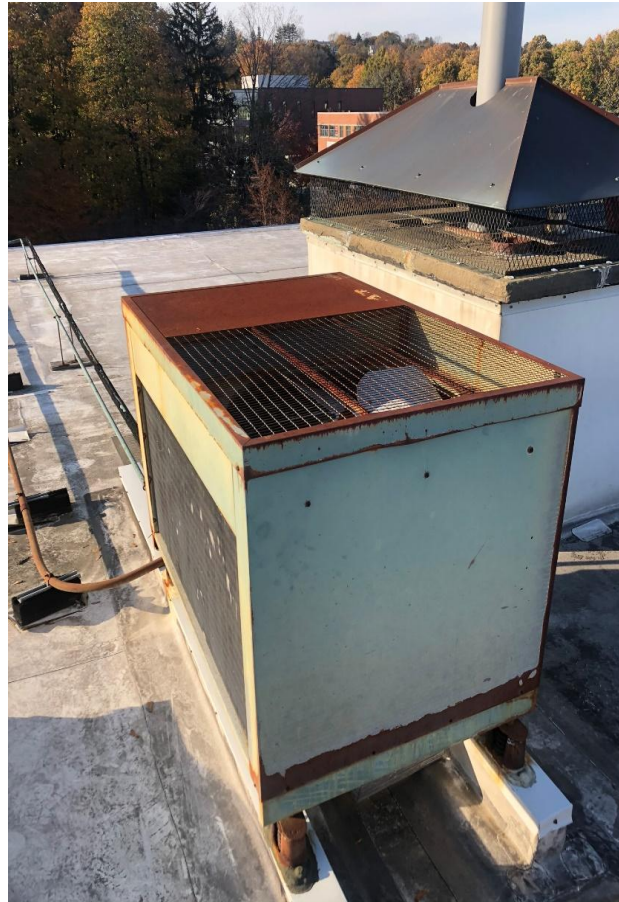
AC Units on roof not designed to carry that load
