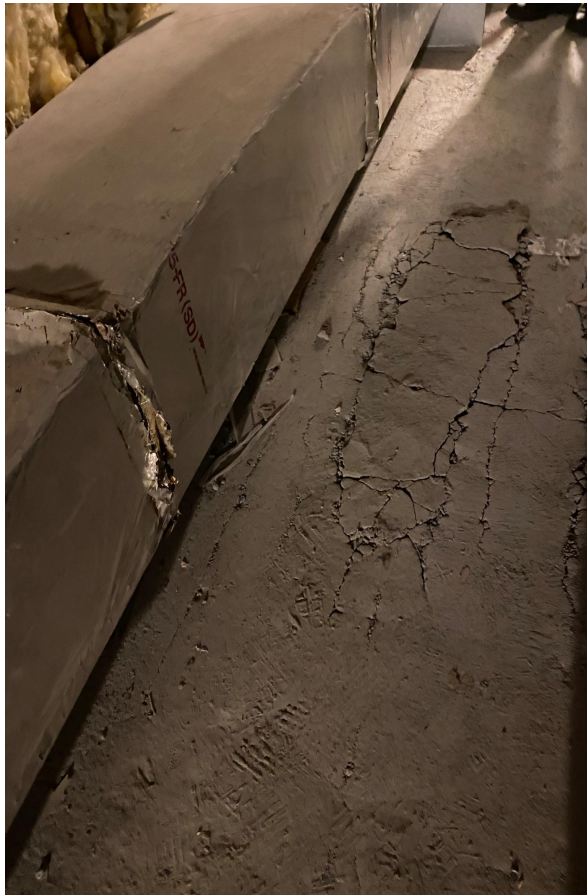
Floor in eaves disintegrating
