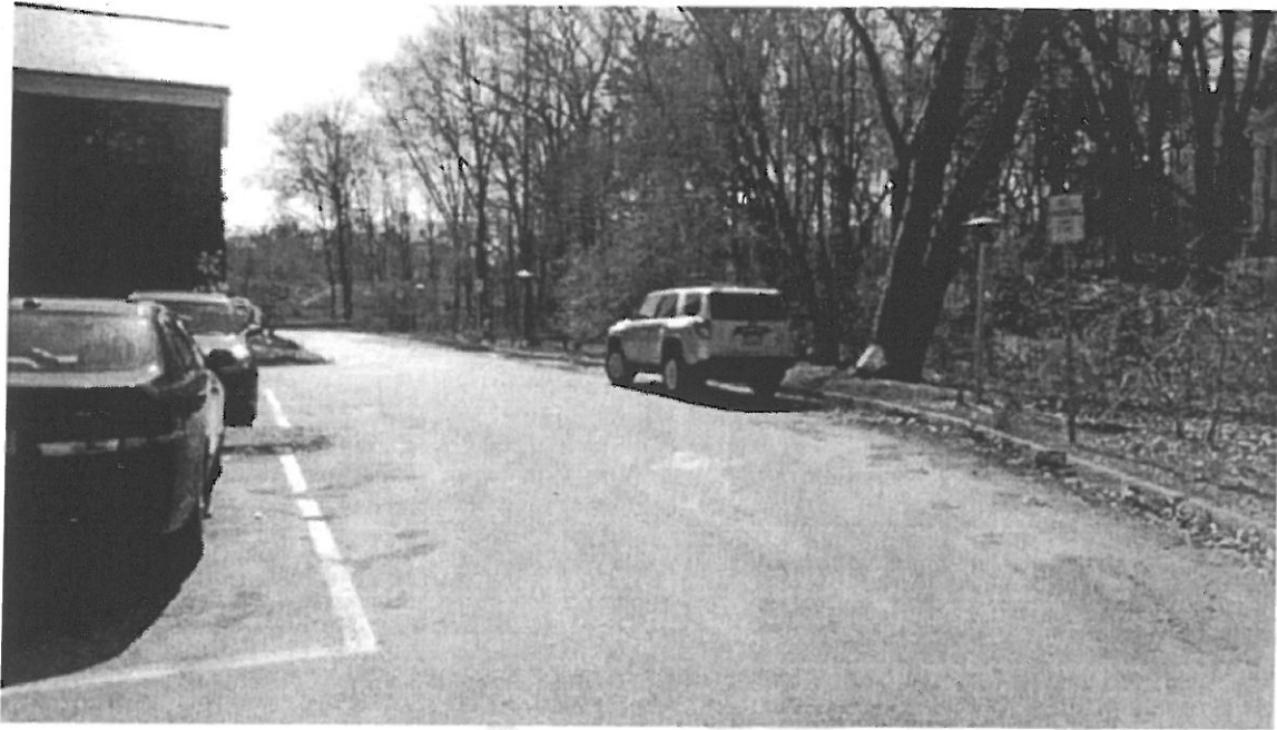
Photo 1. A bituminous curb intercepts sheet flow off the parking lot
