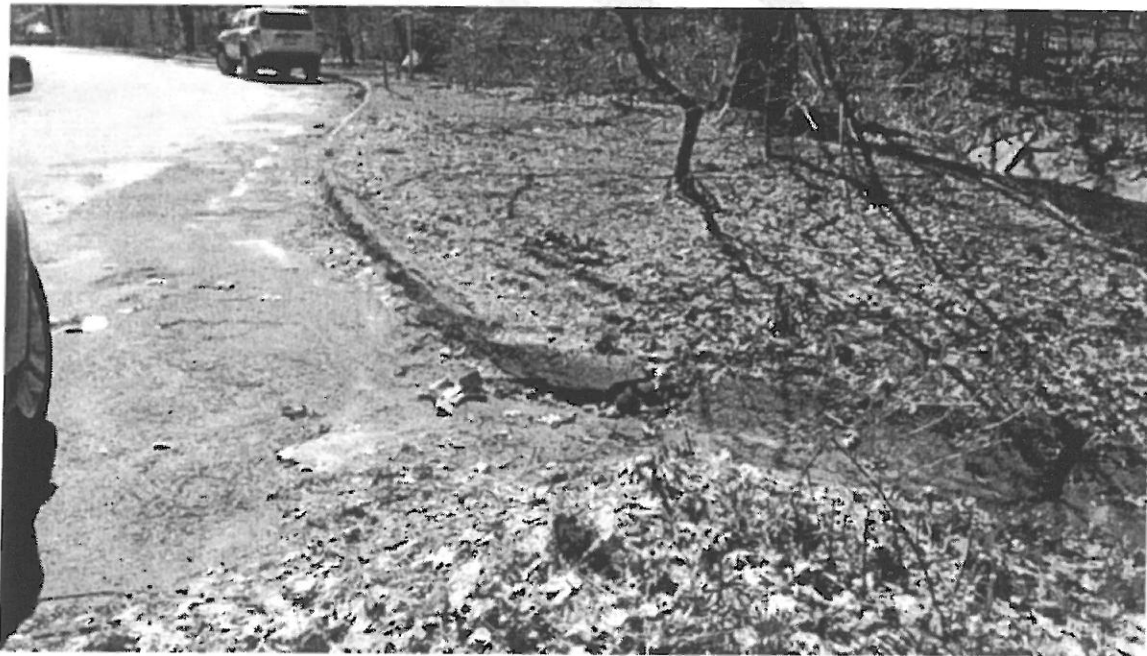
Photo 2. Flow concentrates in a concrete channel at southwest corner and discharges directly to Wellington Brook
